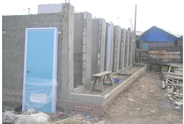
The Public Toilet (After)
